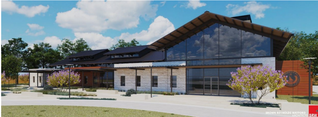
New City Center, Horseshoe Bay City Hall
